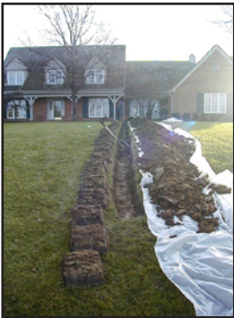
Sod cut out, folded back. Trench dug out on to plastic.
