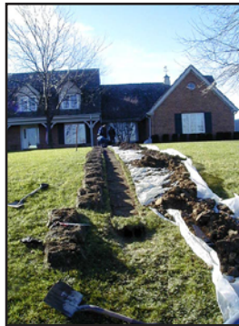
The pipe is installed and dirt is hand tamped.
